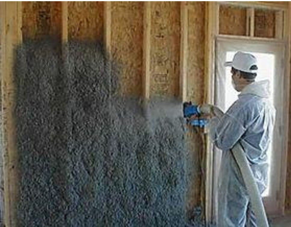
Blown in Cellulose Insulation
