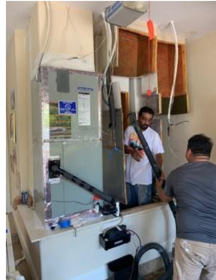
Disassembling and cleaning the AC blower, coils, lining and plenum.
