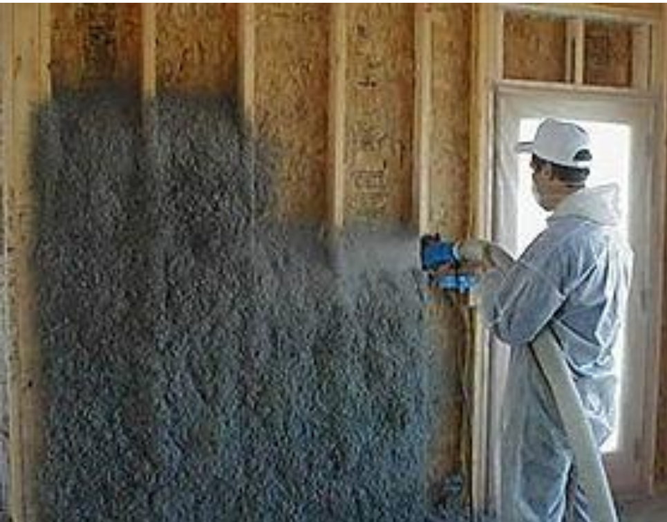
Blown in Cellulose Insulation
