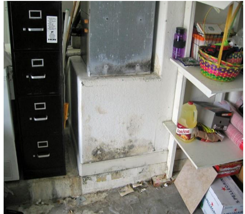
Water damaged AC return air box with mold both outside and inside
